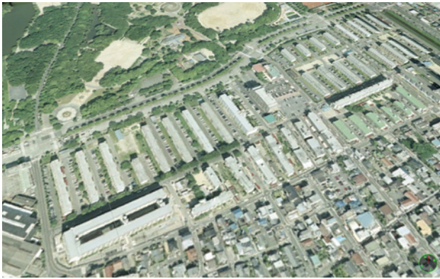
Figure14 Aerial photo of Meijo area, Nagoya city, Japan ( MapCube, 2003)
